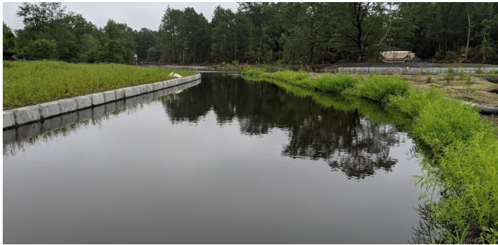
Restoration of Ten Mile River (top) and Mire Brook (bottom)
